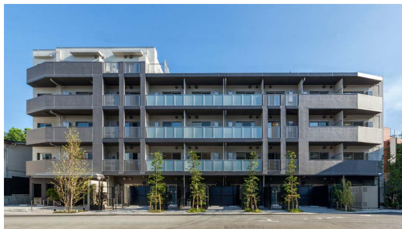
Park Axis Magome Residence
