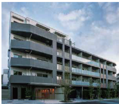
Park Axis Magome Residence
