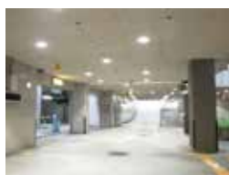
Okawabata Apartment Communities (Parking)
