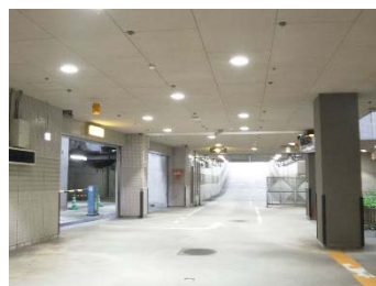
Okawabata Apartment Communities (Parking)
