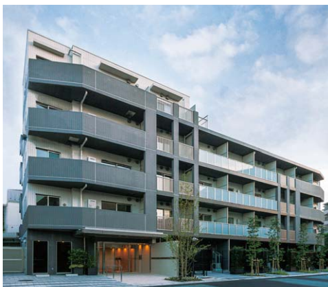
120 Park Axis Magome Residence
